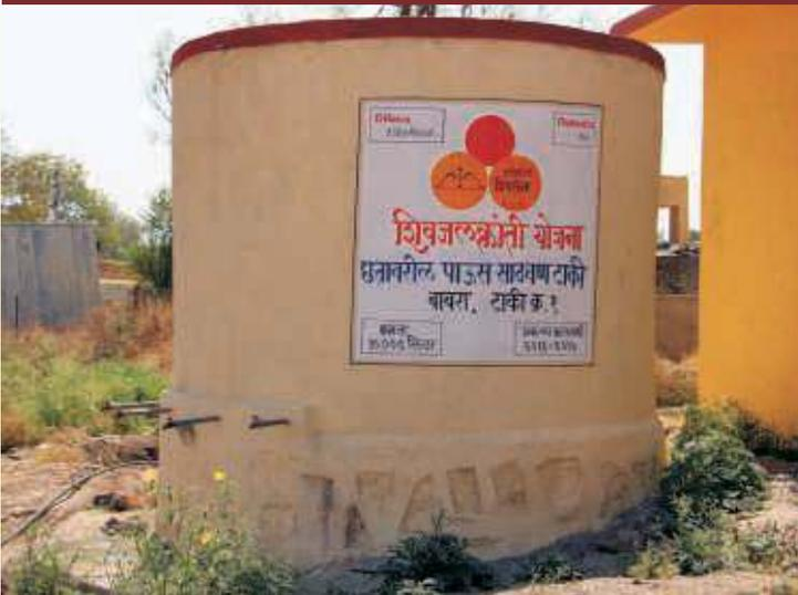
A permanent structure made of ferro cement. The capacity of the tank is 10,000 Litres. The pipes connected to the roof will harvest the rain falling on the rooftop during monsoons and in the lean season it acts as a storage structure. The life of tanks is around 75 years.
