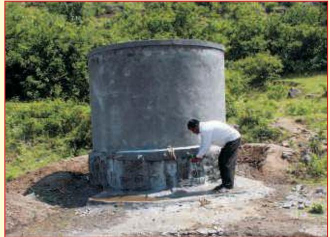
10,000 liter capacity. The tanks are fitted with PVC pipe for roof top water collection with filter arrangement. This structure is mostly used during village festivals to store more amount of water. This has a life of more than 75 years and is cost effective compared to conventional metal or plastic tanks.
