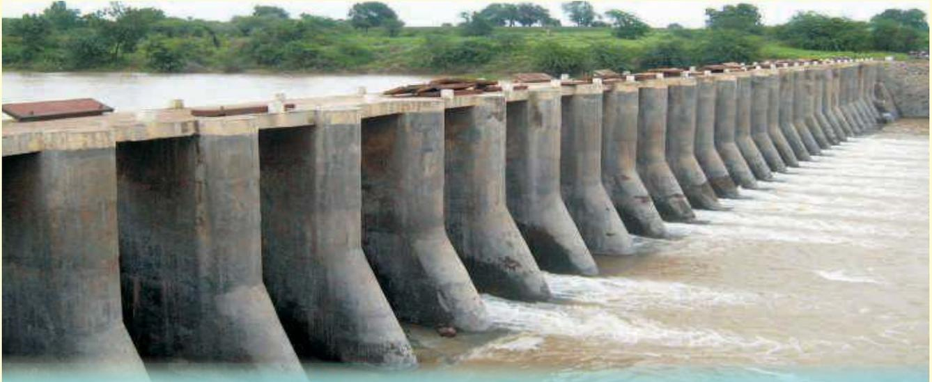
**The repair of K T Weir resulted in the storage of nearly 800 m length back water on its upstream side. The total storage of KT will be 40 TCM which will recharge around 27 wells and 30 bore wells near the banks of Kambli river. The benefit of the construction of wall will not only recharge the wells only in Hivara area but also the benefit will be in Pimparkhed village which nearby Hivara.**
